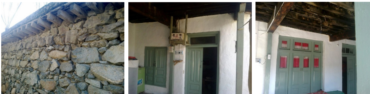
Figure 16. Highlighting Masonry/stone at exterior. Figure 17 and 18. Highlighting mud/cladding at interior
