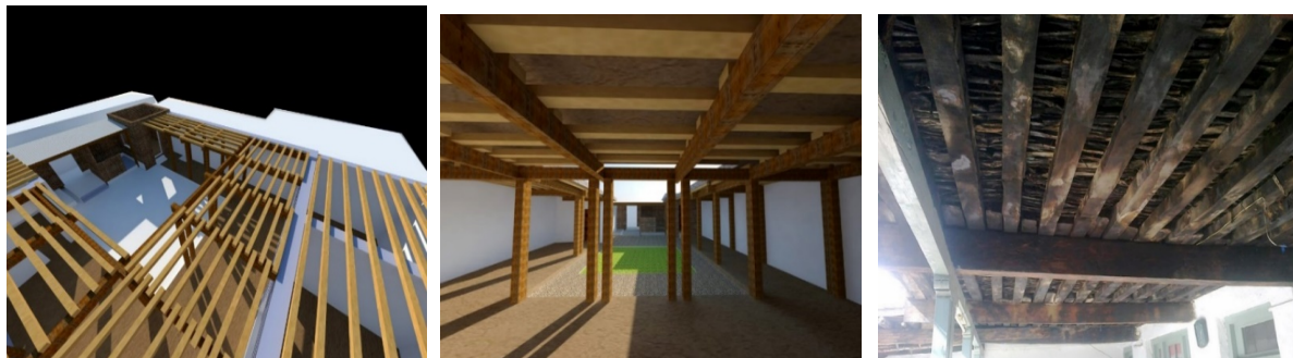
Figure 13. 3D-view highlighting the placement of wood as a structural element Figure 14 and 15. Perspective Highlighting the column and beams as A structural element
